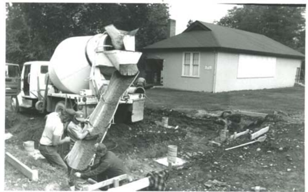
1999.000.051 Pouring foundations for museum cage; 1980s-1990s
